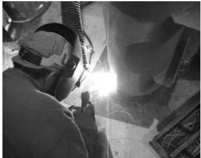
Welding a stanchion (Photo courtesy of Bath Iron Works).
